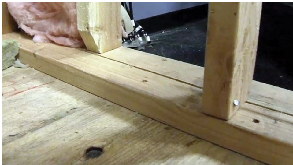
FIGURE 2.2. Wall joists with staggered studs.
